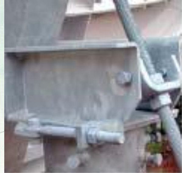
Fine azimuth and elevation adjustments
