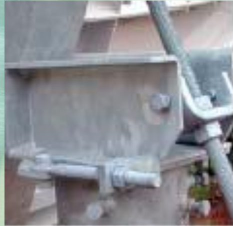
Fine azimuth and elevation adjustments
