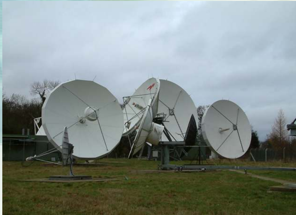
Large earth station antennas
